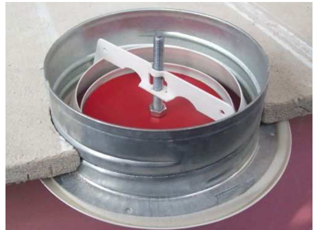
Fire Rated Ceiling Air Valve installed before a fire
